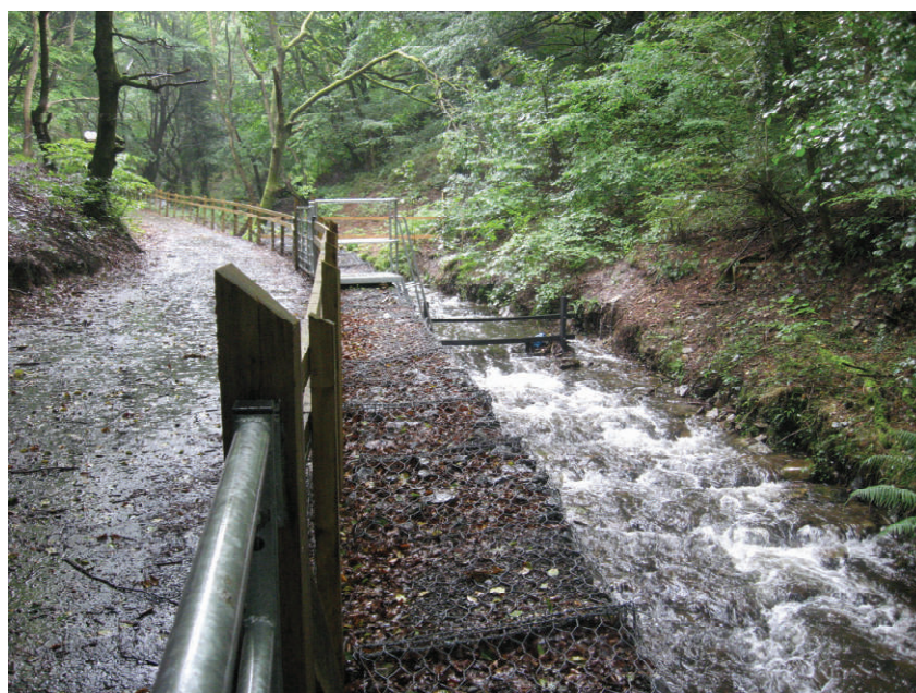
Access track and security fencing adjacent to Nant y Draenog
